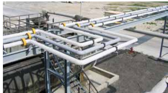
Figure C.6: U-shaped expansion bend
