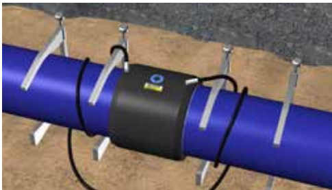
Figure D.21: Connecting the welding machine
