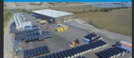
XXL PIPE PRODUCTION FACILITY CHARLESTON, SC/USA
